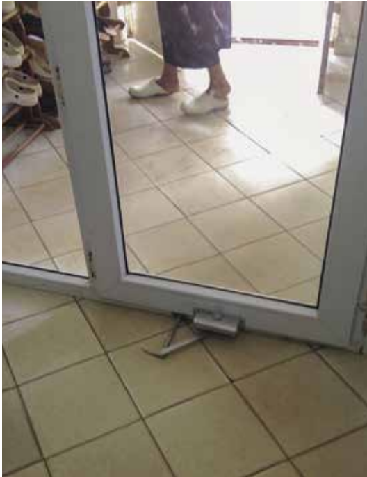
Creative 'bottom-mount' of an automatic door closer: "We did not have enough space above the door..."
